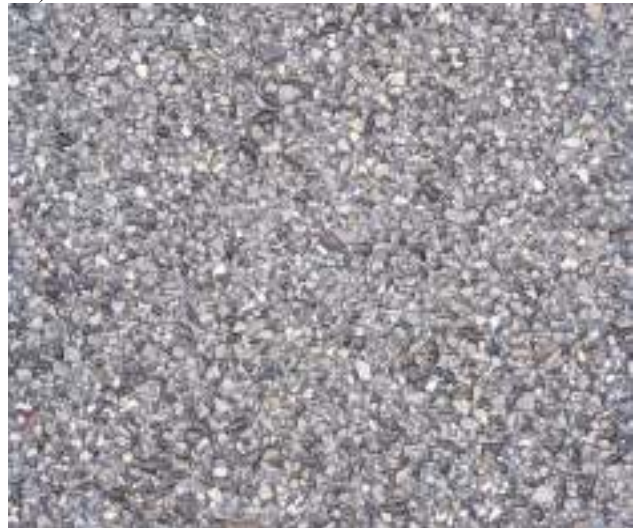
Figure 4 : View of surface texture of SMA after 12 years depending on type of adhesion agent
