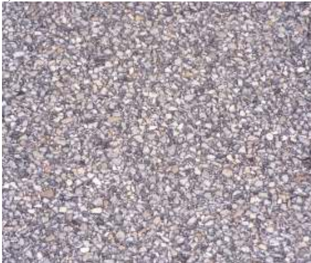
Figure 4 : View of surface texture of SMA after 12 years depending on type of adhesion agent
