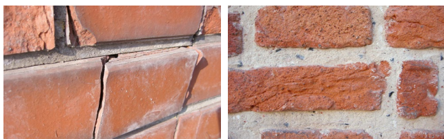
Figure 1. On left: high strength non-lime mortar (thermal and shrinkage movements cause cracking & separation). On right: mortar containing lime (natural movements accommodated without damage).
